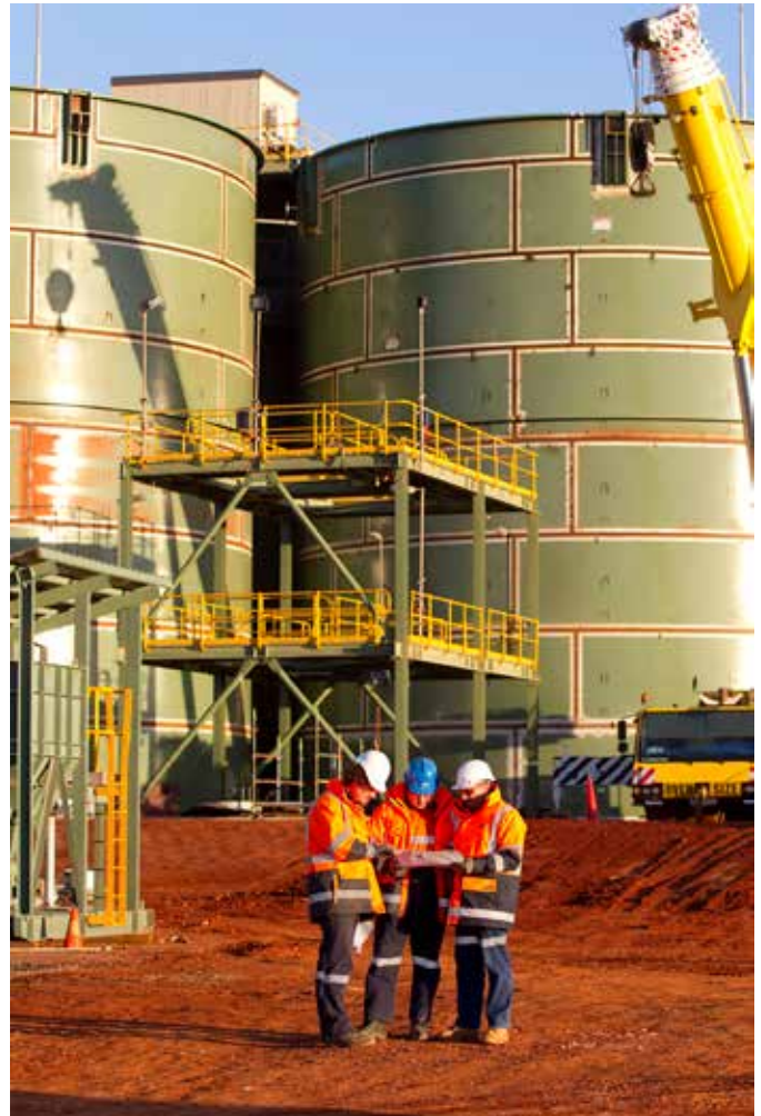
Figure 1: Construction of two additional leaching tanks
